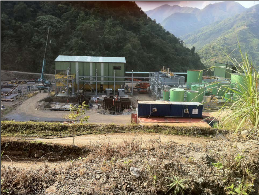
Ban Phuc Concentrator Under Construction
